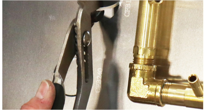
Photo 2: Breaking the Knockouts
