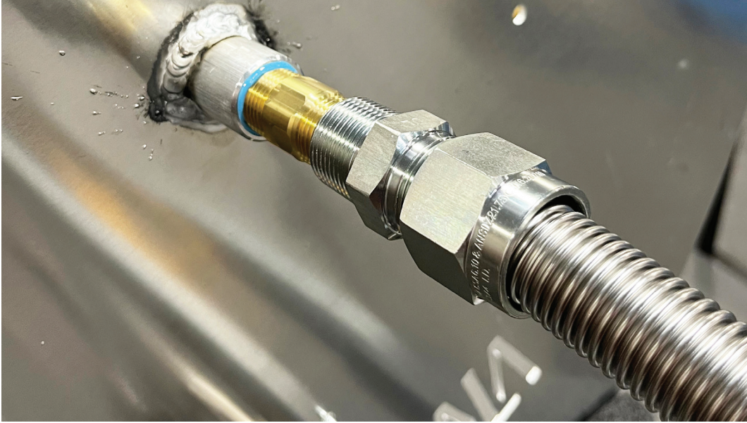
Photo 18: Connecting the Flex Line
